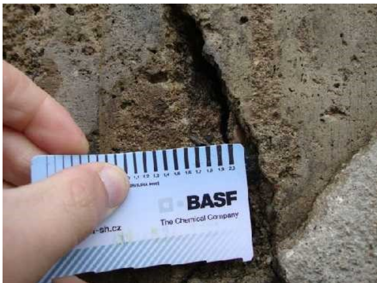
Obr. 16: Detail trhliny.
